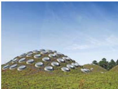
Inside the four-story rainforest dome, visitors can meet live rainforest residents. The 2.5-acre living roof is planted with nine species of native California plants that provide habitat for local wildlife.
